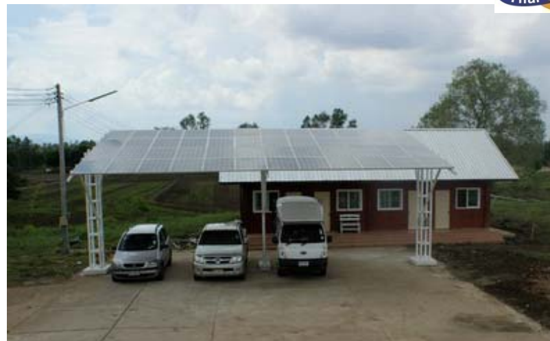
10 kWp, Petchaboon Innovation Co., Ltd., (2010)
