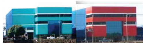
Choknamchai Machining Foam, Machining Laser Cut
